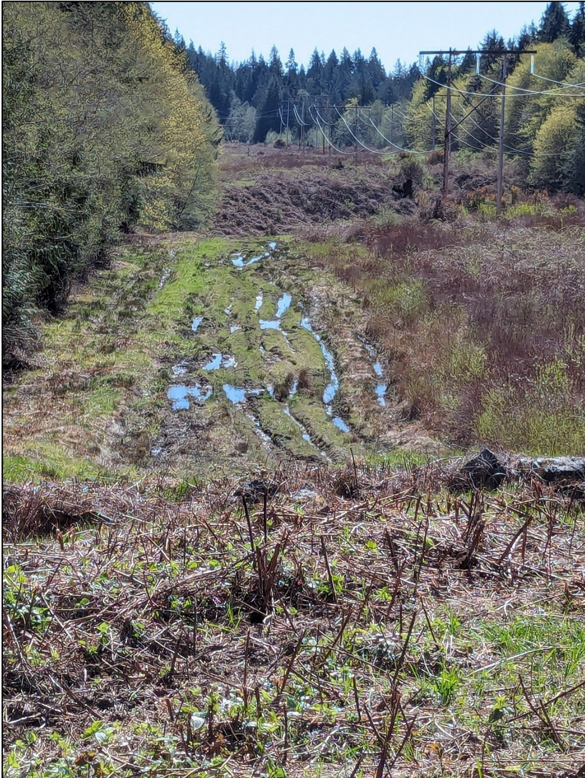
Photo 8: ATV rutting in gas pipeline ROW.
