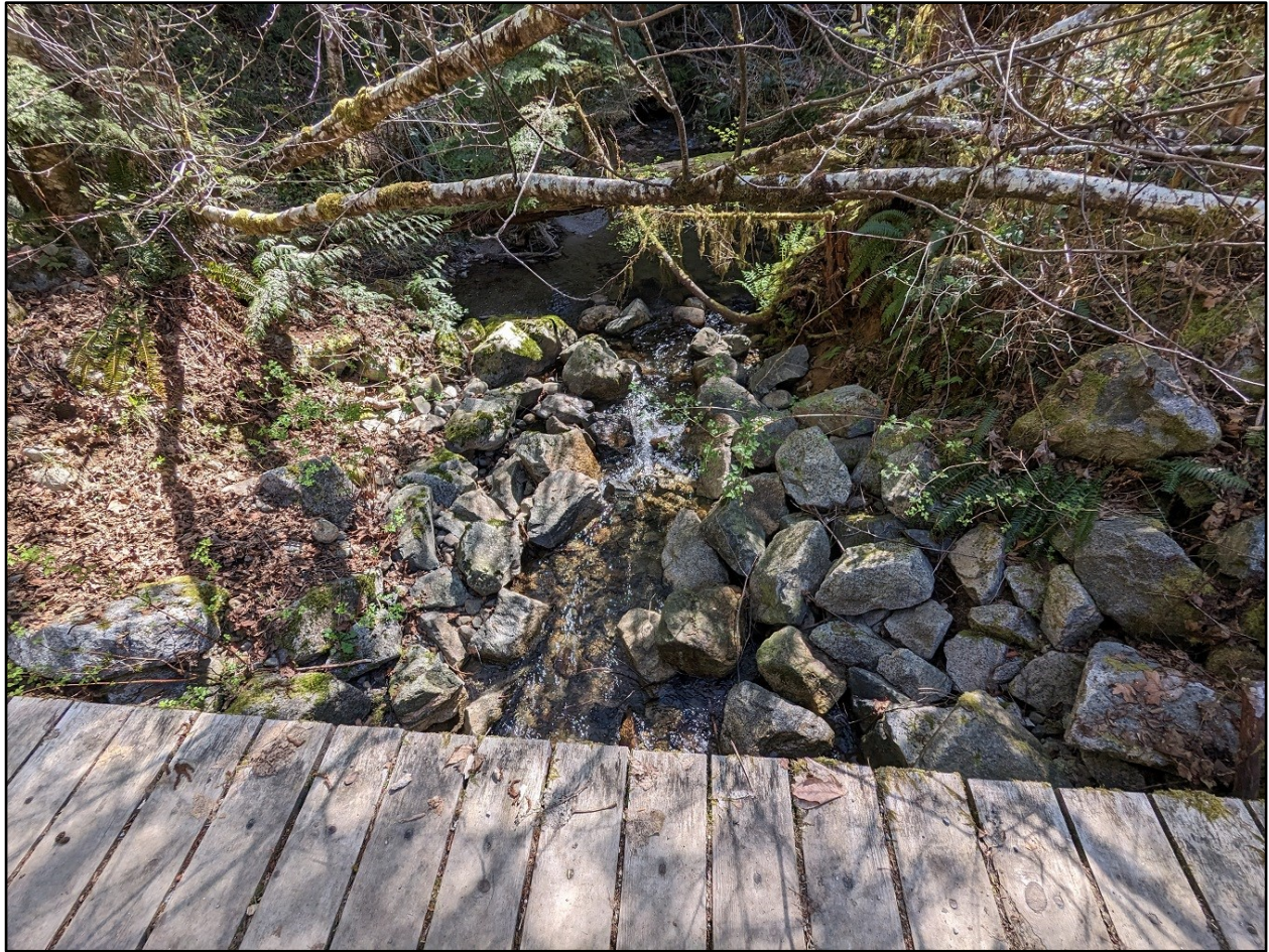
Photo 13: Bridge and coarse rock riprap on mountain bike trail in forest.
