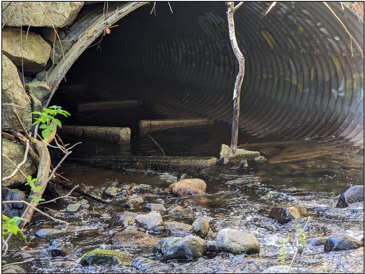
Photo 2: Concrete baffle fish ladder in Highway 101 culvert.
